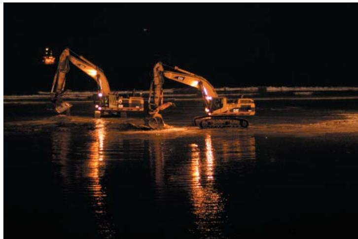
Crews worked through the night during one of the lowest tides of the summer to remove the dam of sand that separated the ocean from the newly created tidal basin. During the dredging of the basin, water from the ocean was pumped in as the sand was being pumped out. When the bridge used by the oil company was completed in July, the inlet opening was scheduled for the next low tide in August. Photos by Mark Bixby.
